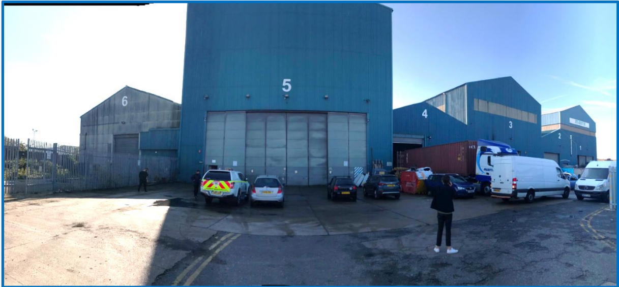
Front of Unit 5
