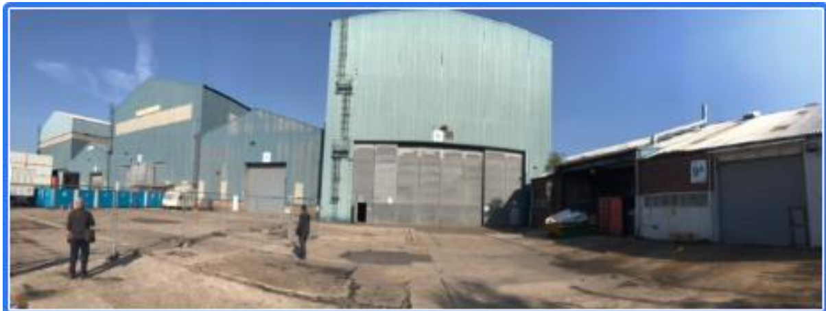
Rear of Unit 5
